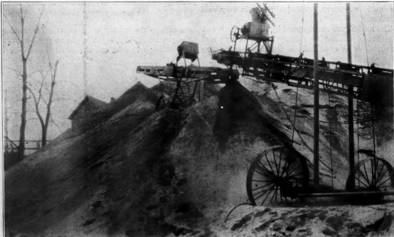
Close Up of Portable Conveyors on Storage Piles
